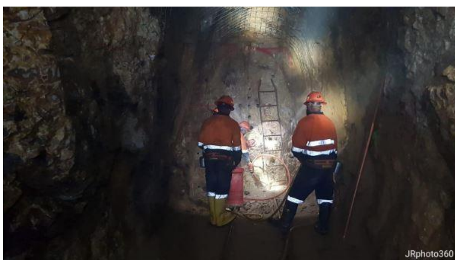
Figure 48: HGZ Mine 1930RL development drive, 2018. (Source : ASX:CGN 19 July 2018)
