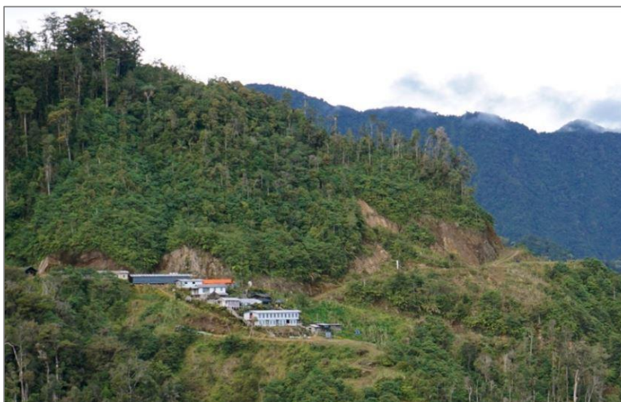
Figure 49: Crater Mountain Minesite office and accommodation 2016. (Source: ASX:CGN 14 July 2017 Crater Gold Investor Update).
