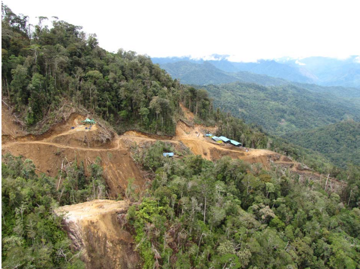
New top camp with NEV 18 (left centre) and drill pad for NEV 19 (left front)
