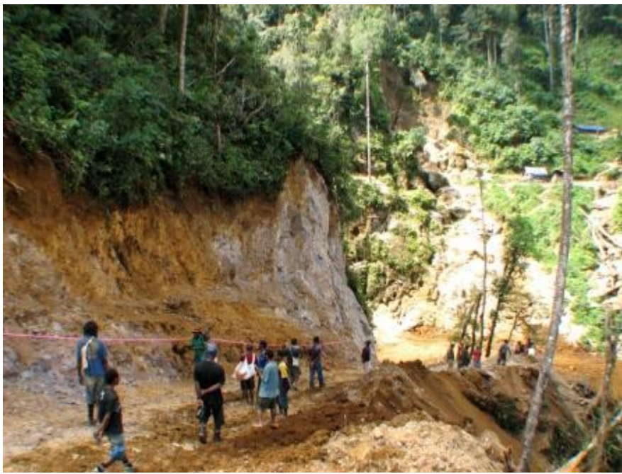
Road cut through spur to base of artisanal mining area in background
